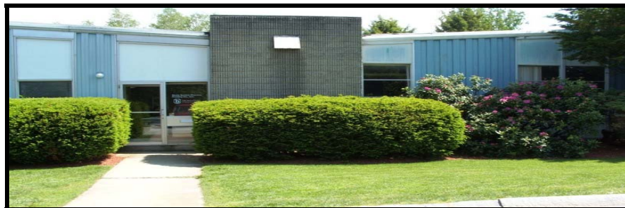
Bovie Screen Building, Bow, NH
